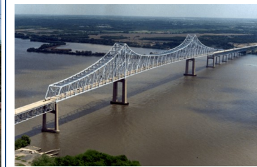
Commodore Barry Bridge over the Delaware in Pennsylvania
