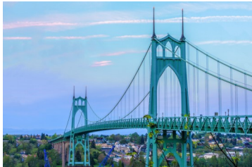
St. John's bridge Portland
